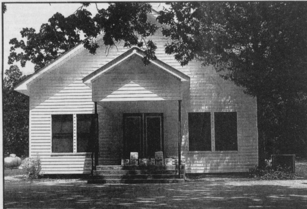
FACE LIFT-the Cuthand Methodist Church has been receiving a face lift. When the congregation could not locate land to build a new church on, it was decided to add onto and improve the one they have. And so it is almost complete. Everyone is welcome to attend, view the new improvements and share in worship. (Staff Photo Nancy Brown)
