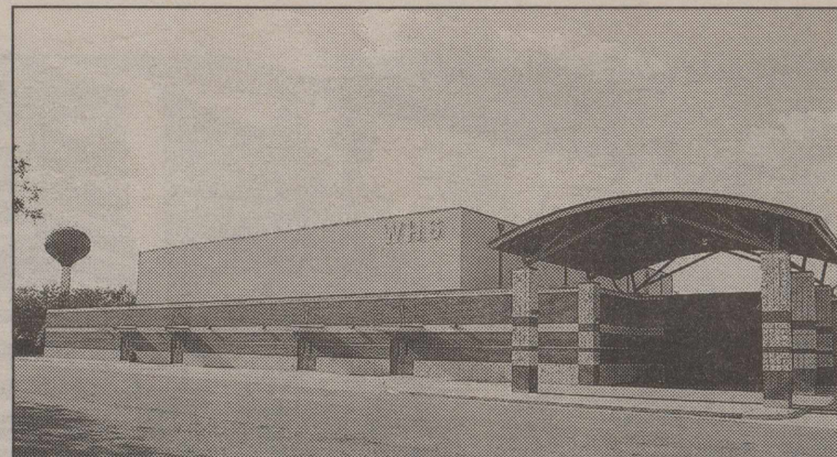
Winters High School Special Events Center, built in 2010.
