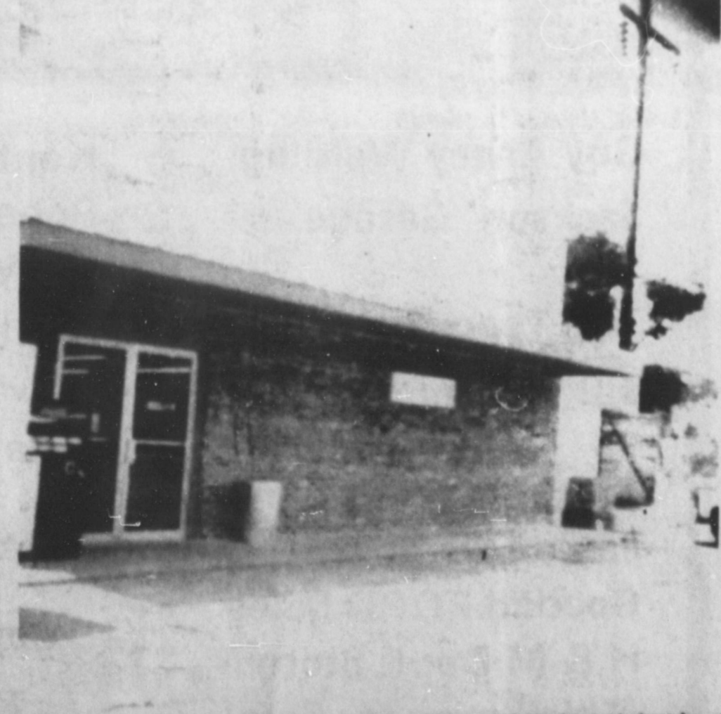
Jayton food store has recently undergone a face lifting, with the front windows being taken out, and a new brick front put in. It really enhances the looks of the place. Chronicle photo.
