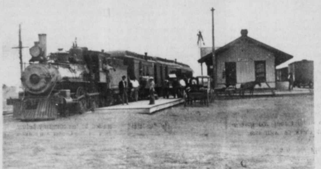
FORGOTTEN HISTORY--Here is a picture made in 1912 of a train at the Jayton Station. At that time the passenger traffic was heavy, as people rode the train to Spur, did their shopping, and then caught it back to Jayton again. Photo courtesy of Adolphus Moreland.
