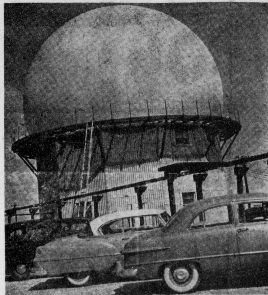
The radar antenna is contained in this giant, air-inflated rubber ball, revolving in perfect freedom. The rubber covering is to protect the antenna from damage by the weather, and keeps down corrosion that might otherwise affect its usefulness.
