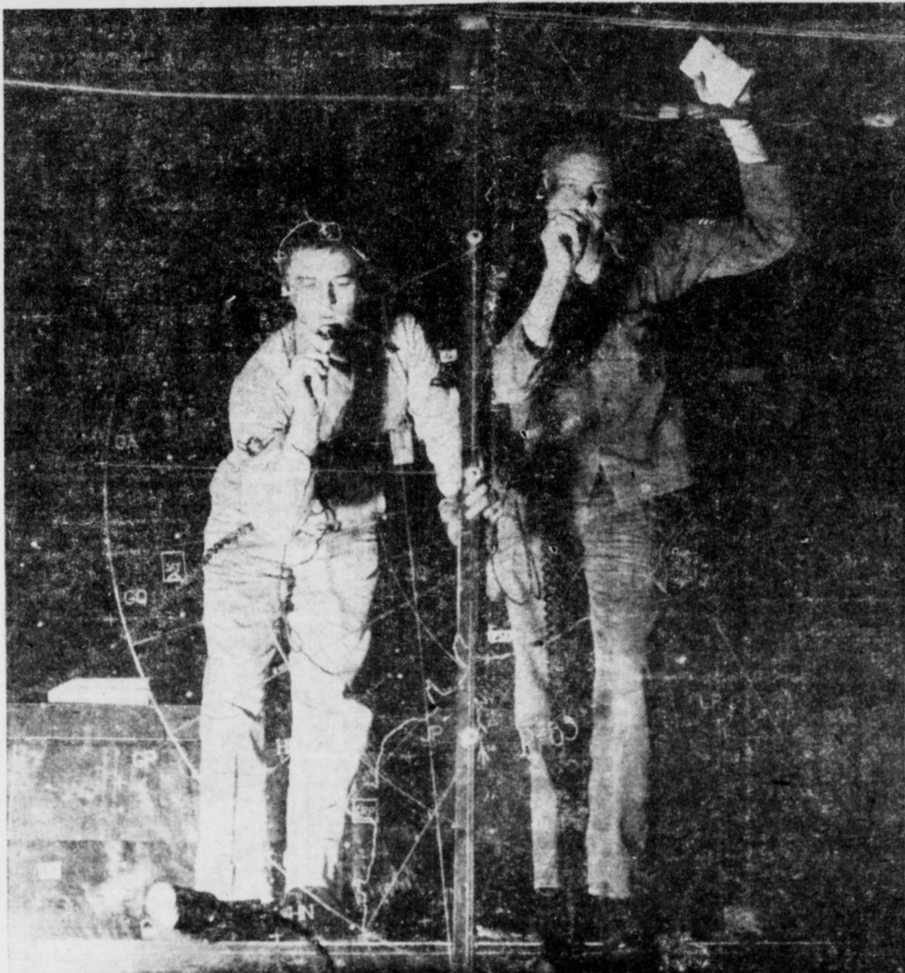
This giant sheet of plexiglass is the main point of interest in the Aircraft Warning Station at Ellington Air Force base, and the real heart of the installation. The men shown here write backwards, so that their figures can be read from the front of the plastic sheet. On this they indicate by numbers, arrows, and letters, the position of any aircraft observed by the giant radar antenna, which is a part of the station. This information, collected by a crew which sits in front of the plexiglass, is relayed to these markers, who then set it down, so that still other men can see the whole picture at a glance, and relay the information thus collected to headquarters at Oklahoma City. From there, in condensed form, it goes to command headquarters in Kansas City, to be passed on immediately to the heart of the system in Colorado, which receives similar data from all over the North American continent.
