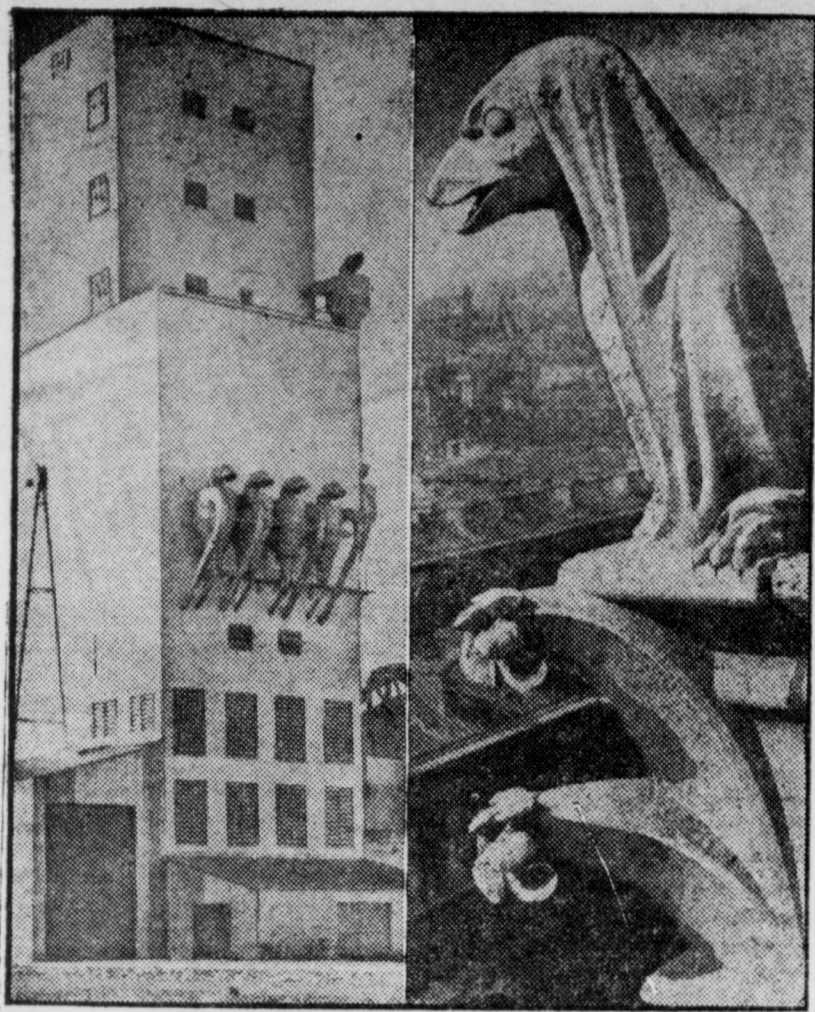
20TH CENTURY GARGOYLES — Gargoyle, at right, looks across the centuries from his rampart atop Notre Dame Cathedral, Paris, at its 1955 counterparts on outer wall of the Farmers' Rice Growers Cooperative processing plant at West Sacramento, Calif. These present-day mechanisms help to rid plant of dust and moisture, even as the gargoyles serve to top outlets for water runoff on roofs of medieval structures.
