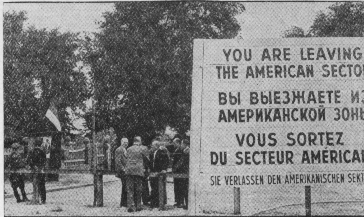
BRIDGING THE GAP —A severe water shortage in Berlin's Neukolin district momentarily washed away East-West barriers as officials from both sides met to discuss the problem. An earlier agreement on mutual water deliveries made possible this meeting on a bridge linking the American and Soviet sectors. Note East Berlin police "guarding" the meeting.
