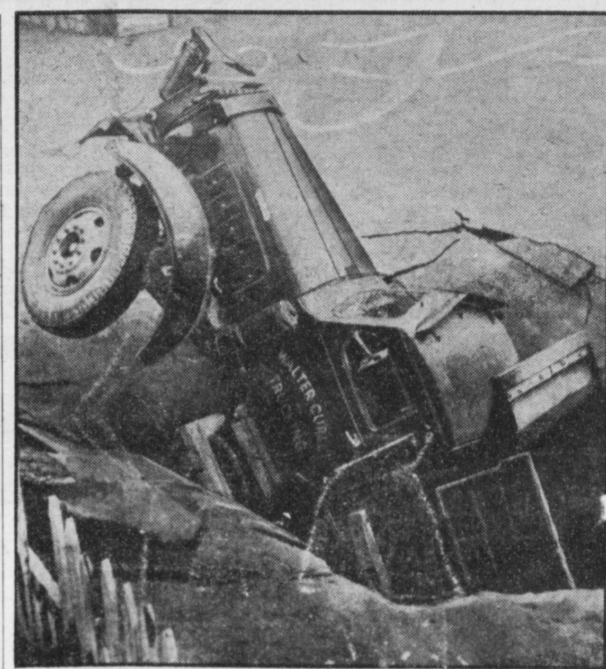
BACKING DOWN —Boston truck driver Walter Curley backed his seven-ton truck on a bridge, suddenly realized he was backing down to a lower level. Investigation showed the rear wheels had passed over a weak spot in the bridge and the heavily loaded vehicle dipped toward bottom. Curley, surprised and dazed, climbed from the cab uninjured.
