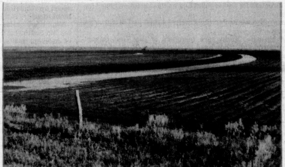
The construction of terraces and diversions is an excellent way to control and stop erosion on rolling land and sloping cropland. With terraces and diversions, rainwater is channeled across the field to a suitable outlet such as a grass waterway or pond. Through this channeling action, water is transported across the field and isn't allowed to cut down across the field, stopping erosion and the development of gullies.
