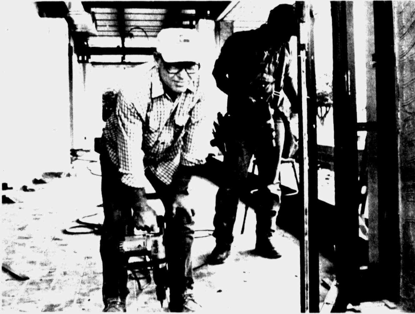
GLASS MEN — David Brooks and Todd Taylor, both of Lubbock, are shown installing glasswork in the entrance section of the First Baptist Church's
