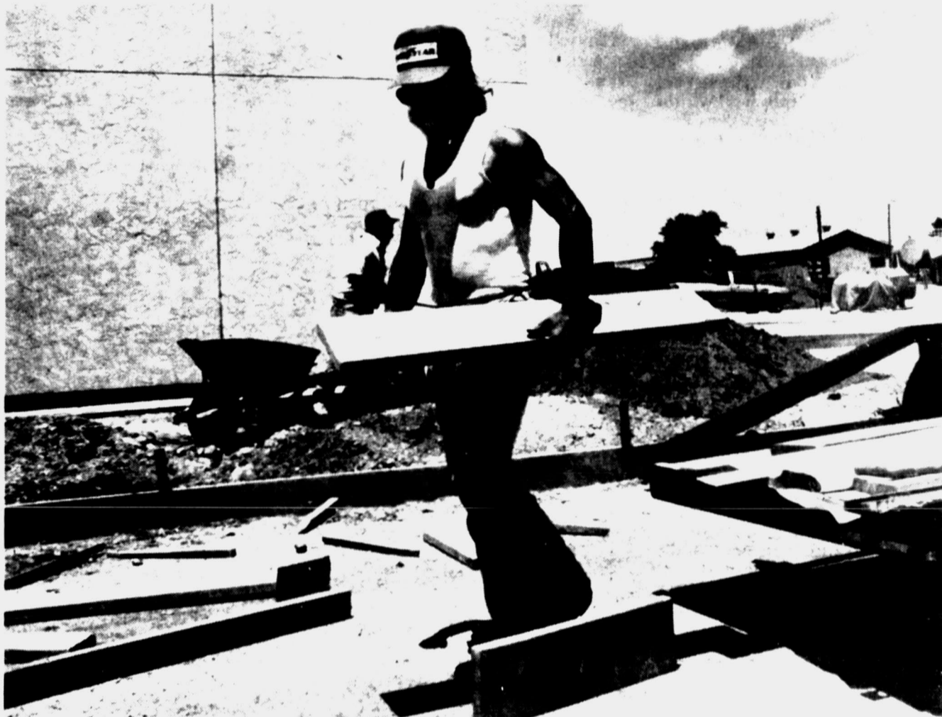
CONCRETE WORK — Angel Gomez of Lubbock was cutting lumber to use in concrete forms at the First Baptist Church's new multi-purpose building, which the general contractor, Sunwest
