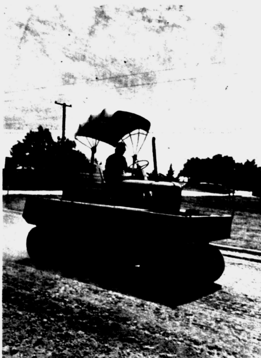
SMOOTH, SMOOTHER, SMOOTHEST — County road and bridge crews are creating a smooth caliche surface in the Towle Park Rd. renovation project. The work marks the first complete resurfacing of the roadway since it was built in 1952. (SDN Staff Photo)
