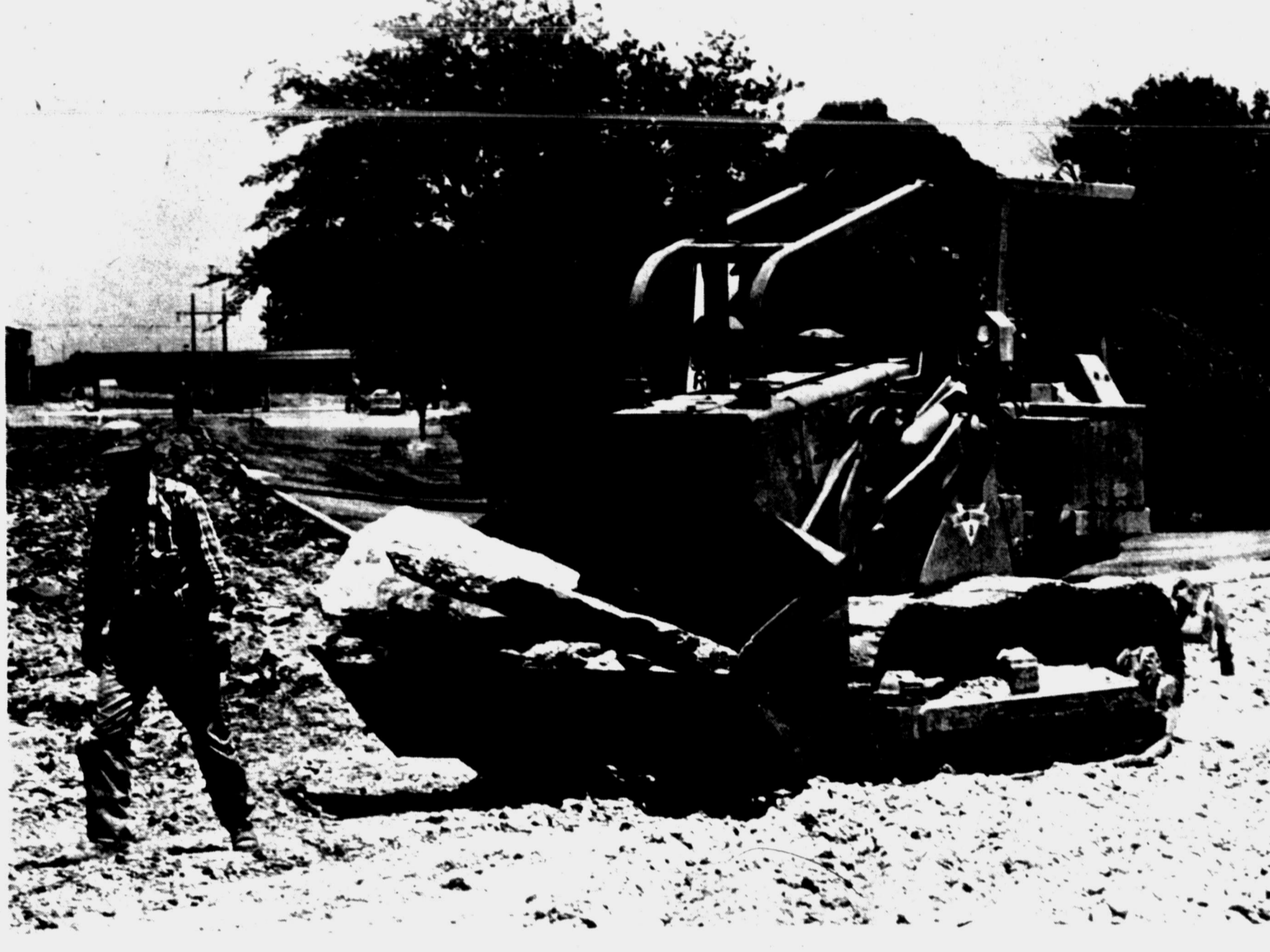
TEARING IT UP — A.P. Smith, left, of commissioner's Pct. 1 and Ronnie Hines of Pct. 3 were tearing up asphalt and concrete last week on the county-owned Towle Park Road, which is being completely reworked for the first time in its 37-year history. (SDN Staff Photo)
