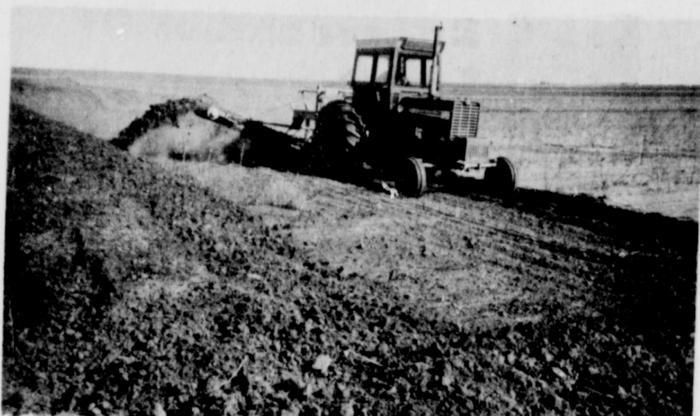
TERRACE WORK —Malcolm Tunnell is shown above just completing work on a system of parallel terraces on the Rudy Derhoff farm, which is operated by Troy Bradshaw. Bradshaw farmed following the contour lines laid out by the U.S. Soil Conservation Service last year in preparation for building the terraces this spring.
