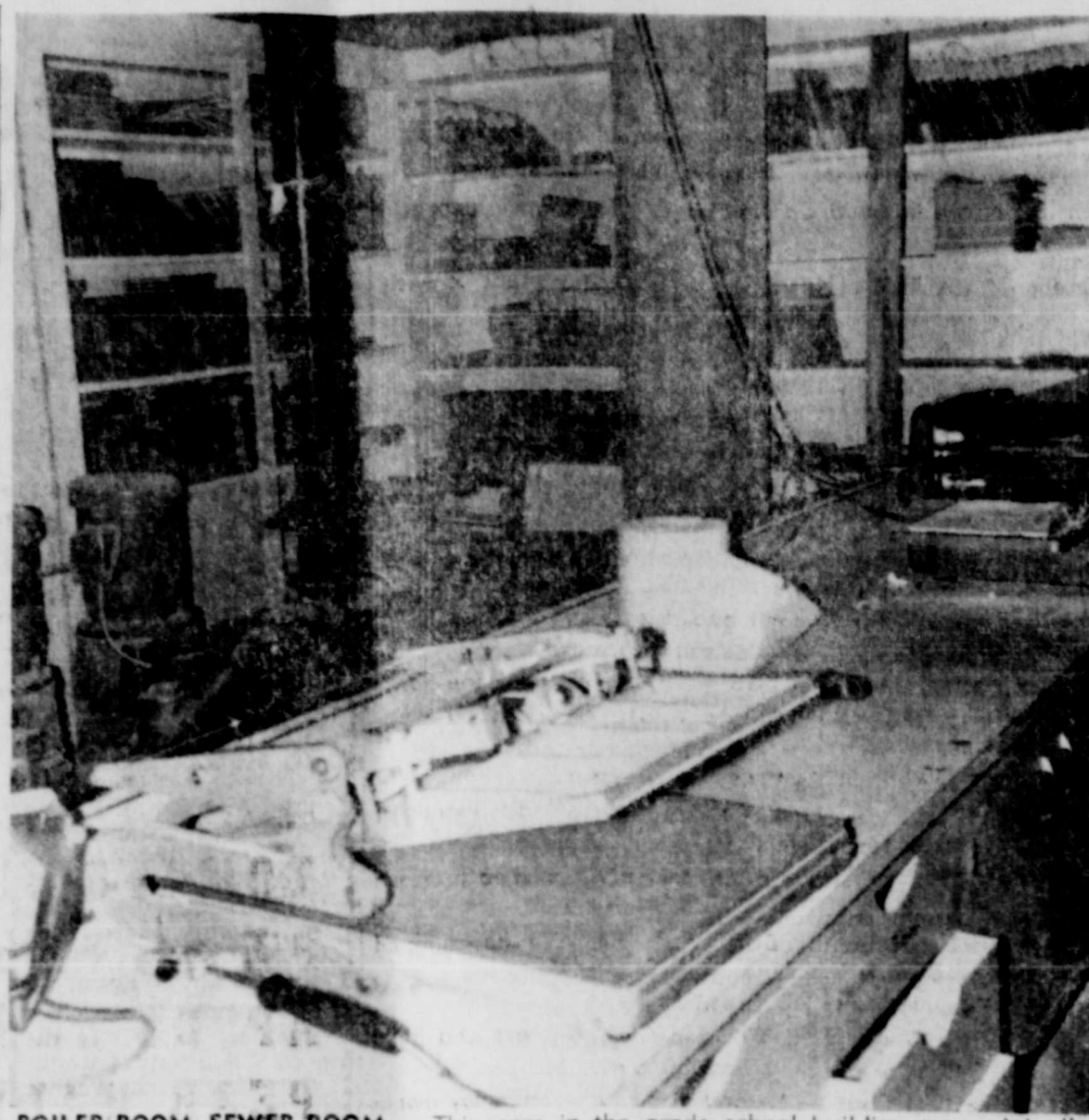
BOILER ROOM, SEWER ROOM — This room in the grade school building was originally the boiler room and janitor's closet. Now it is a book storage room, mimeograph room, you name - it room. It is next to a kindergarten room next fall.
