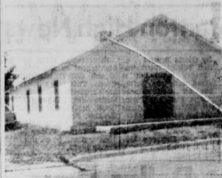
ONE ROOM SCHOOL HOUSE —Actually, this building is a church, but the school must rent it in order to have enough class rooms. Mrs. Elmore teaches one fourth grade class here.
