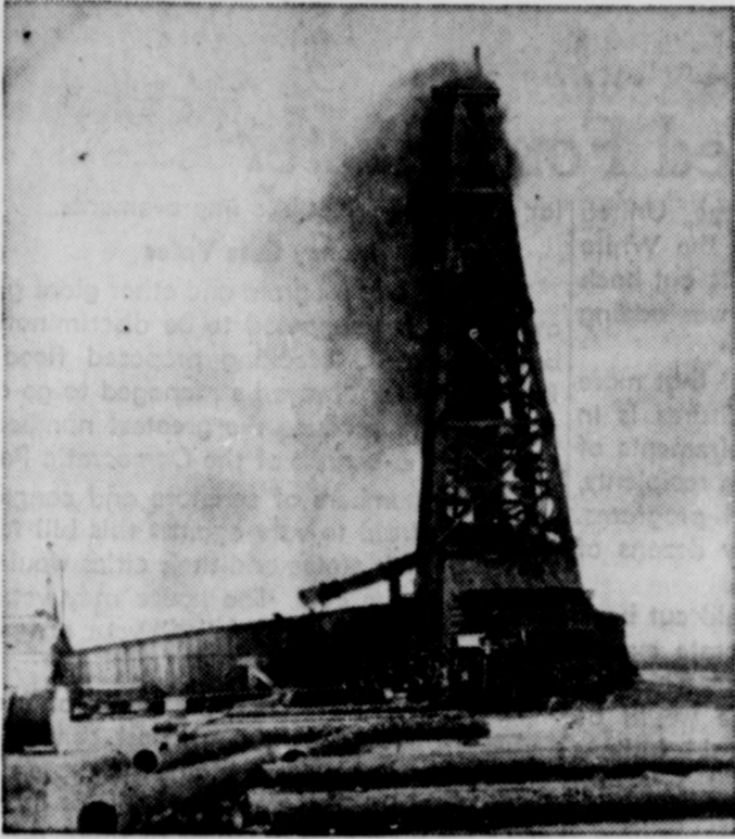
SANTA RITA, 1923 — This well drilled on University of Texas land in West Texas opened up the Big Lake field, May 28, 1923, from a depth of 3,028 feet, and drew attention to the now famous Permian Basin oil province and put the first "oil money" in the University Permanent Fund, which now holds more than $447 million from royalties, rentals and bonuses.
