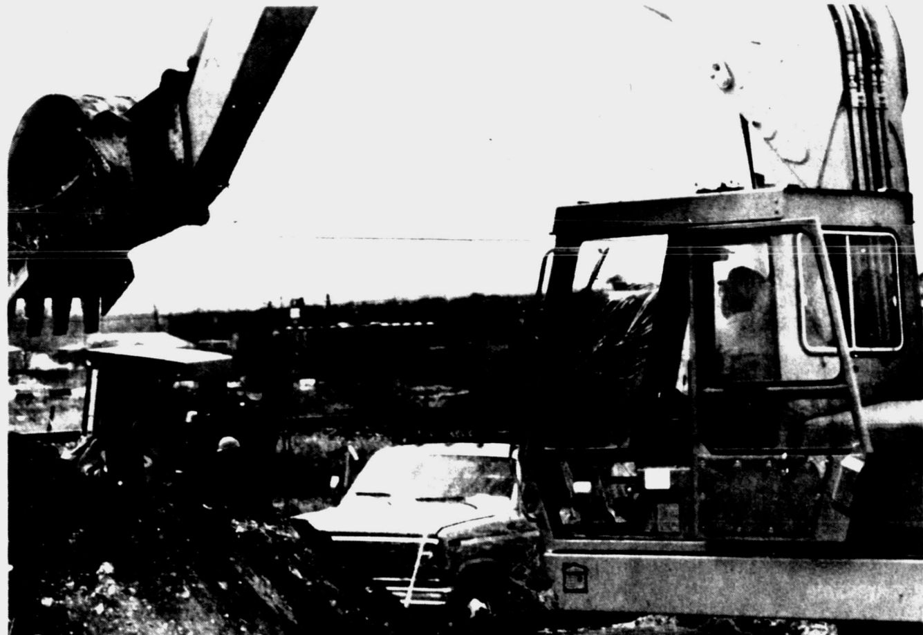
TDC WORK ONGOING — Workmen were busy project to lay utility lines to the TDC Daniel Unit. work began on a lift station at that site, part of the (SDN Staff Photo)
