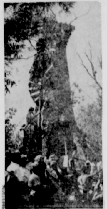
The 44' tall swamp tree slide on Skull Island at Six Flags Over Texas is built around what once was a fire escape at a dormitory at the University of Texas. Students climb the spiral staircase around the outside of the tree and slide down the long corker-type slide inside.
