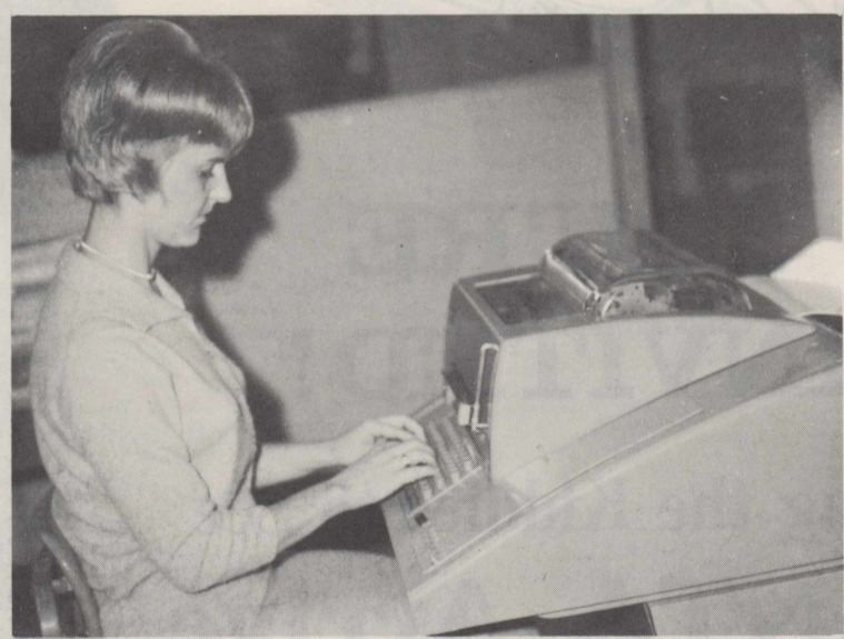
REMOTE UNIT — Mrs. Loretta Downing, inventory manager, inputs an issue request to the UNIVAC from a remote device in Base Supply. Her directions move by telephone wire from a typewriter-like keyboard.
