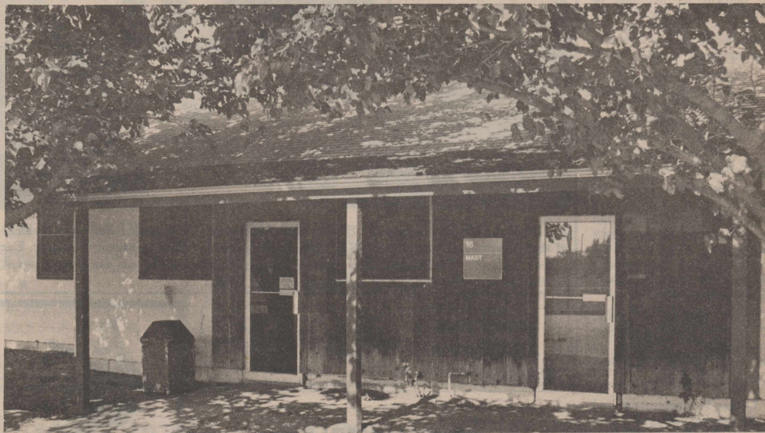
The MAST center, Bldg. 16
