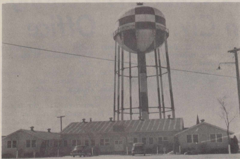
Shown above is Headquarters, Bldg. T-1. Here is located the executive offices which carry on the Wing's paper work. Directly behind Headquarters is Reese's notable landmark—its large water tower.
