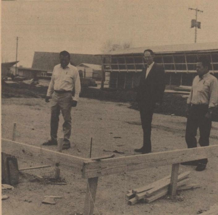
The corner is set; a new building is being built at Forrest Lumber Company. Henry Hicks, manager, Jerry Shipley, assistant manager, and Juan Ramirez observe the new building site. The new 180 foot long, 50 foot wide warehouse will have 16 foot side walls with a 25 foot high peak at the roof. The new 9000 sq. ft. building will be located on the present property at 201 S.W. Ave. B.
