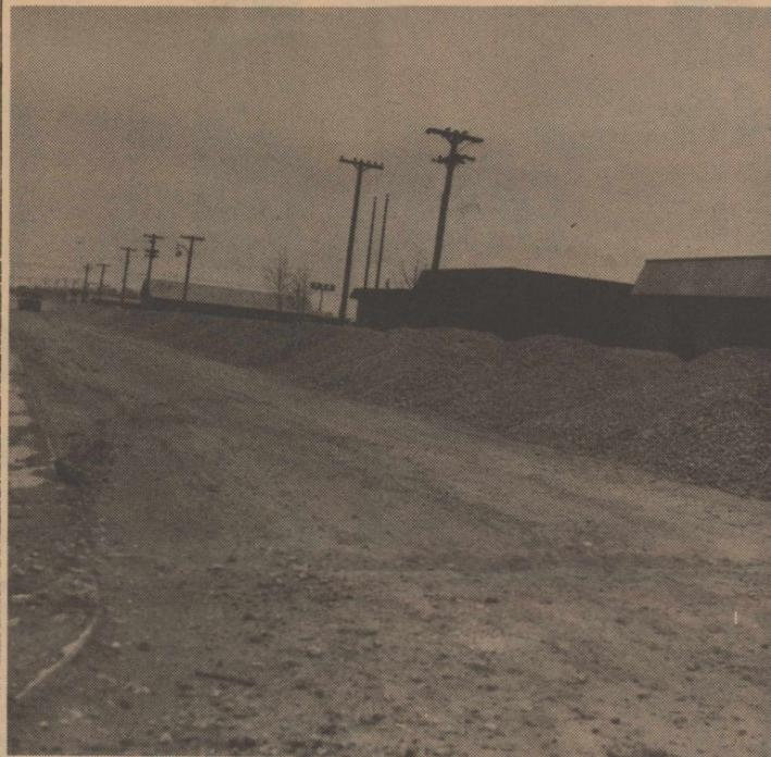
MORE BLOCKS ARE READY FOR PAVING - the curbs are run and the caliche loads out on N. W. Ave. B. The M. S. Doss Scout Center can be seen in the background.
