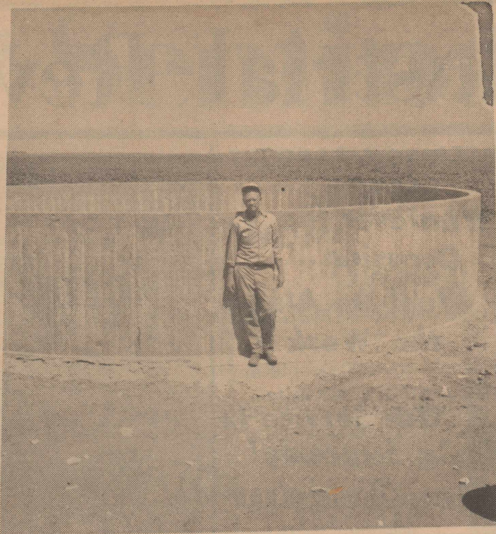
IN THE ABOVE PHOTO, DWIGHT SMITH OF LOOP, TEXAS STANDS NEAR THE TANK HE HAS INSTALLED AS PART OF HIS IRRIGATION WATER GATHERING SYSTEM. IRRIGATION WATER WILL BE PUMPED OPEN DISCHARGE INTO THE TANK FROM SEVERAL WELLS. A BOOSTER PUMP AND MOTOR THEN PUMPS THE WATER UNDER PRESSURE INTO THE UNDERGROUND IRRIGATION PIPELINE. WITH THIS TYPE OF COLLECTION SYSTEM WATER CAN BE PUMPED MORE ECONOMICALY THAN IF ALL THE WELLS ARE PUMPED UNDER PRESSURE. THIS TYPE SYSTEM IS ESPECIALLY GOOD WHERE SEVERAL SMALL PRODUCING WELLS CAN BE USED TO PROVIDE ONE GOOD SOURCE OF WATER.
