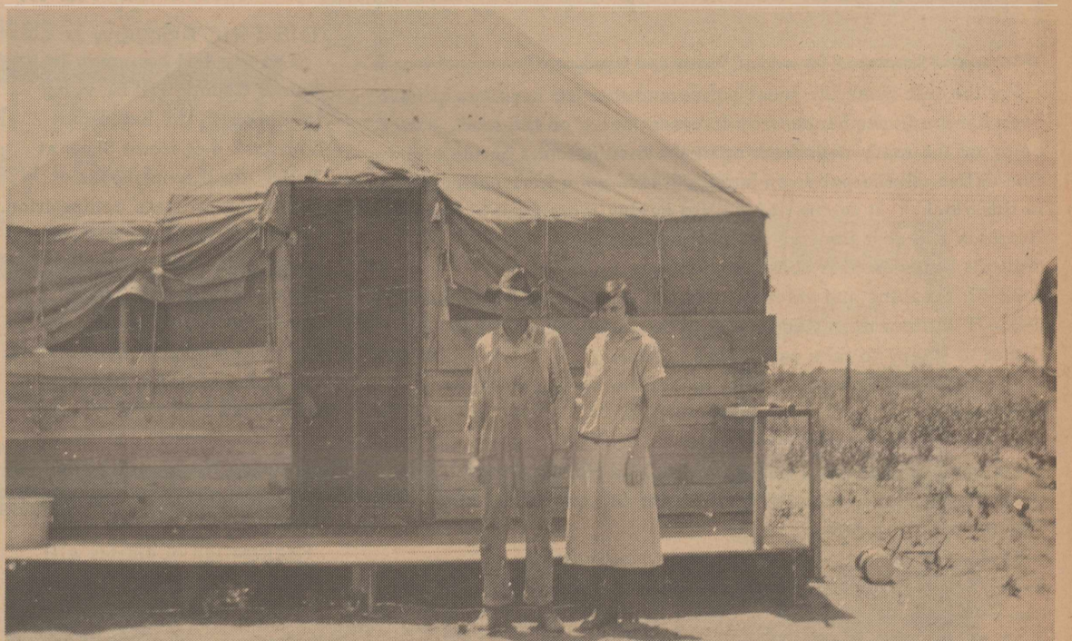
The cook shack on location at the first oil well drilled in Gaines County. Dee Coker worked on the rig and Eunice Coker ran the kitchen. Please note the No. 3 wash tub setting on the front porch of the floored tent. This type structure was known as half of a tent. The flaps are simply rolled up to make the windows. The portion between the wood and the top of the tent was screen wire.
