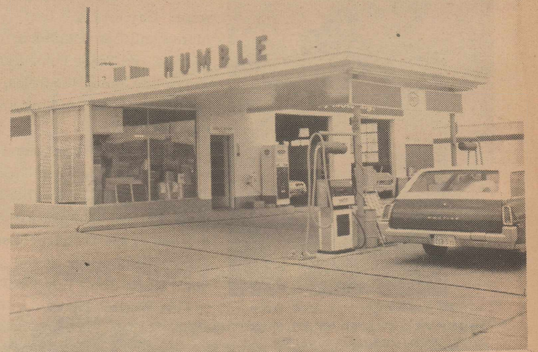
Benson's Enco Service Station, 201 E. Ave A
