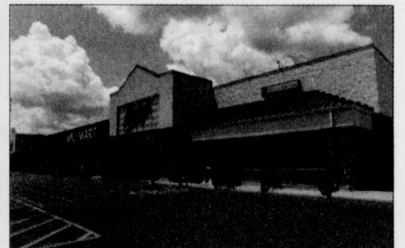
Courtesy Photo THE NEW WAL-MART Supercenter will be more than 200,000 square feet and located on the southwest corner of 4th Street and Avenue Q.
