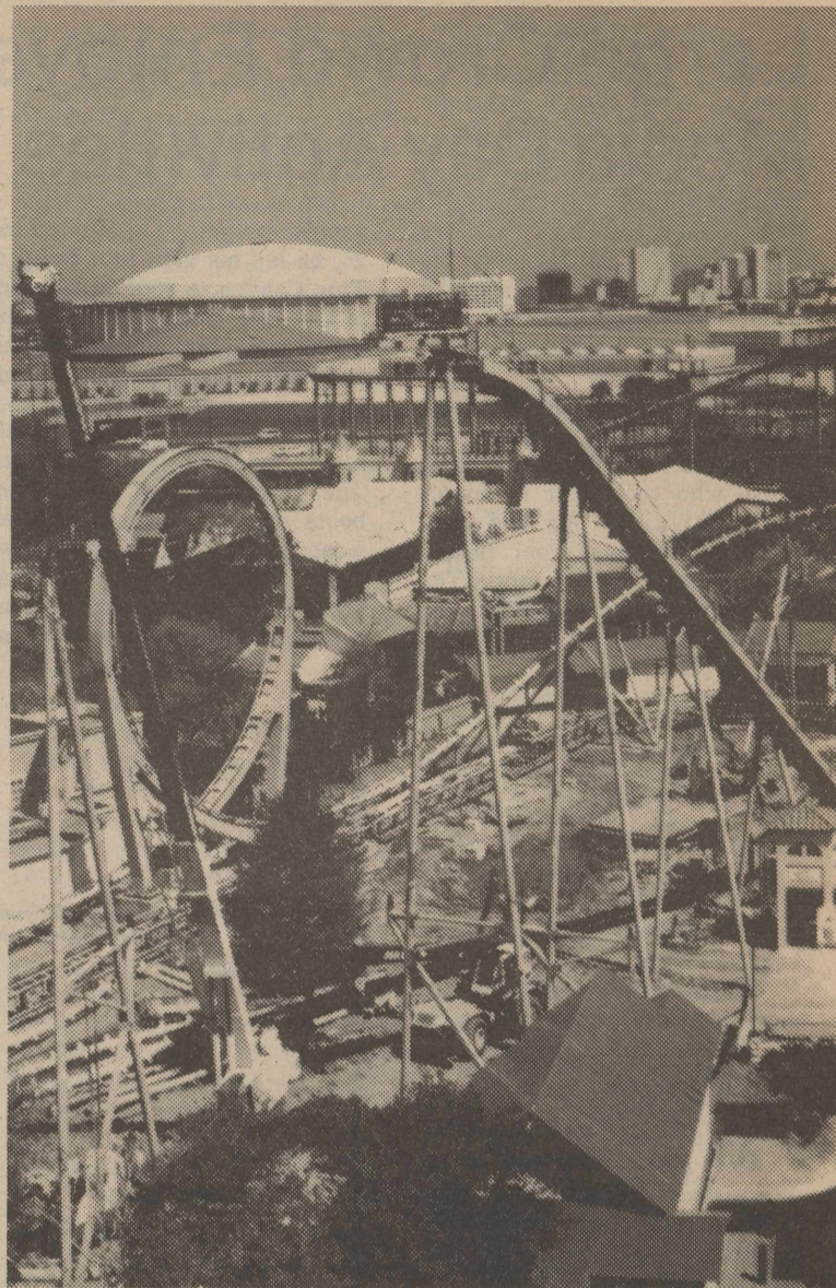
Coaster enthusiasts get ready! Construction on the Viper, AstroWorld's new steel loop coaster, nears completion. Workers continue to lay the 1,968 feet of track that will make up the ride. The Viper, which features a 360-degree loop, corkscrew turns and a 60-foot long tunnel, is scheduled to open this month. AstroWorld, currently open weekends in Houston, is a member of the Six Flags family.
