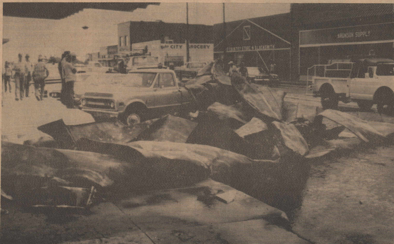
This is what Main Street in Quitaque looked like following the brief storm that hit town two weeks ago. The blow was of brief duration but winds were reported to have reached 90 miles per hour. The debris shown in the photo came from the roof of the garage located across the street from Caprock Home Center. Two pickups and an automobile were covered. Members of the Quitaque Fire Department quickly cleared the street.
