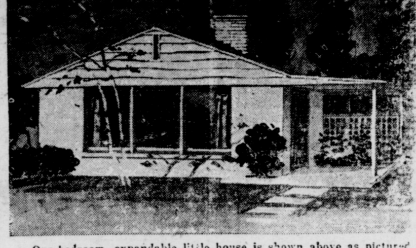
One-bedroom, expendable little house is shown above as pictured in the May issue of Good Housekeeping magazine. Home unit is only 29 by 22 feet, and should cost from $1,900 to $5,000 to build. Other rooms can be added later.
