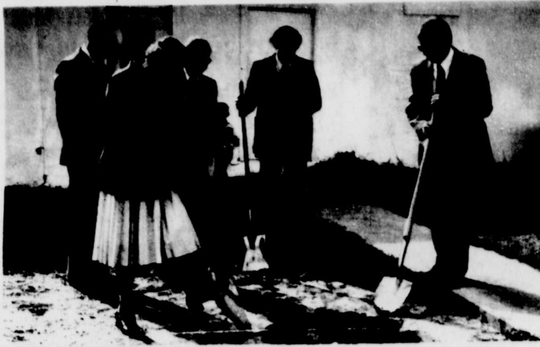
BREAKING GROUND- The members of Calvary Baptist Church, 1800 Conrad Hilton in Cisco are shown in the above photo breaking ground for the new building that will be built behind the sanctuary. Shown left to right are Wayne Webb deacon, Ruby Dunlap charter member, James Harris deacon, James Laird deacon and Ronnie Shackelford pastor. The boy standing in the background is Justin Clement who attends Calvary with his family.
