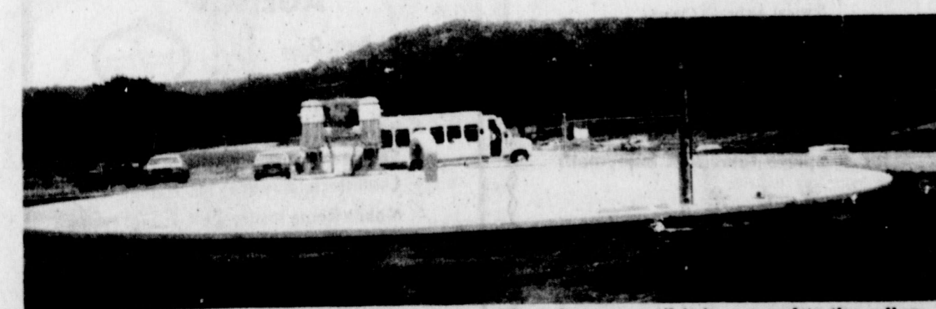
THE CLEAR WELL at Lake Cisco's water filtration system is visible in the above photo. It holds 100,000 gallons of water and stores the
