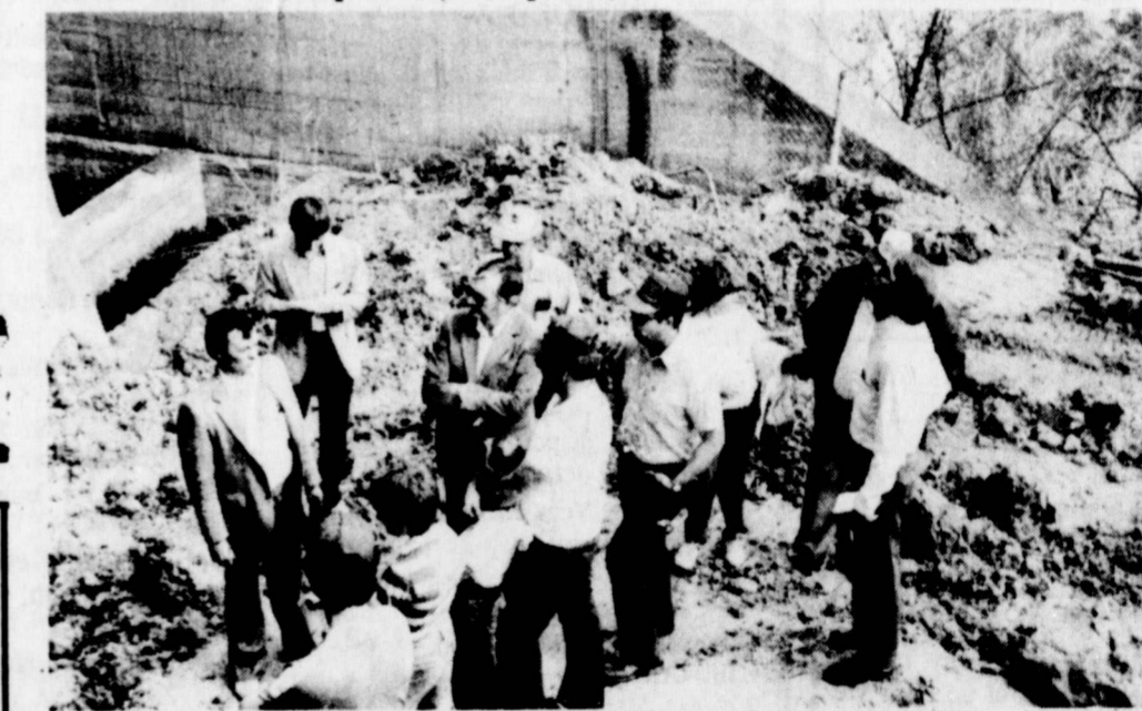
KEN MARTIN, city engineering representative from Jacob & Martin showed those on Saturday's tour where the new water system will tie into the raw water line below the dam. (staff photo)
