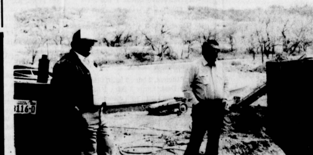
REPRESENTATIVES of Ben Sira Company, the contractors for the project, were also present for the tour Saturday morning. They are Joe Purcell, job superintendent, and Wimpy Jones, project foreman. (staff photo)
