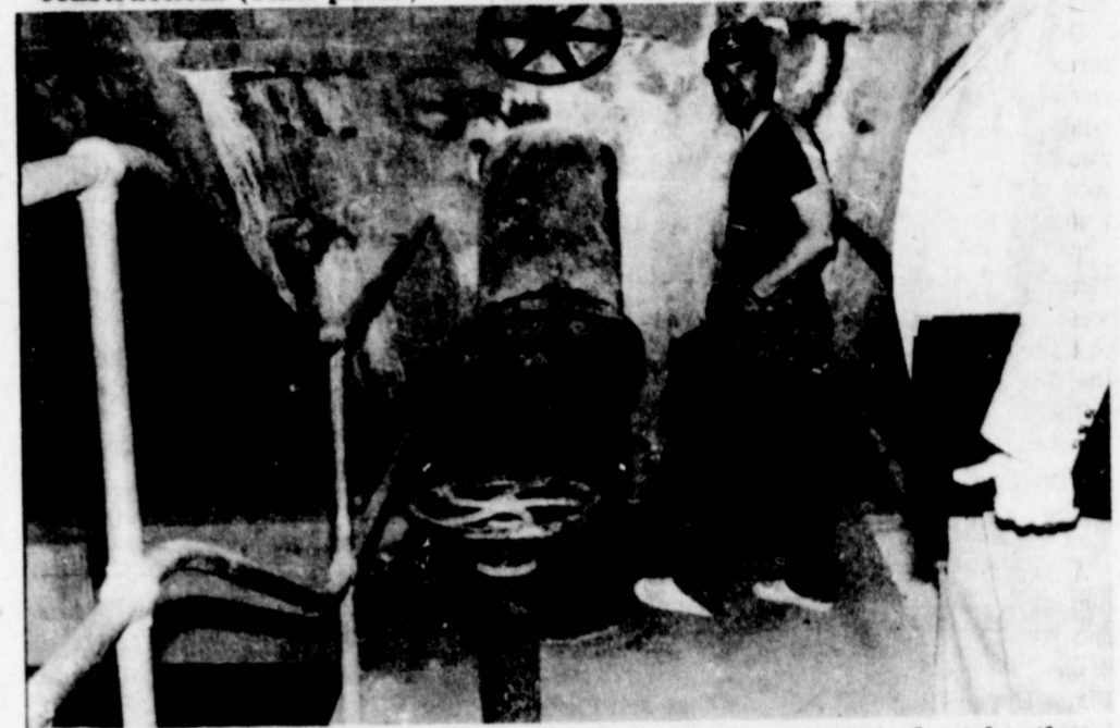
THE CONSTRUCTION site of the new water treatment plant for the City of Cisco is located near the dam at Lake Cisco. Holding tanks and the old pump station are visible in the photograph above taken during Saturday's tour of the facility. (staff photo)
