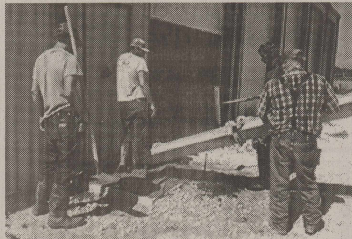
Pouring Concrete in front of the doors at the firehouse
