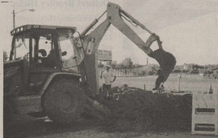
City maintenance crews working on the broken water line.
