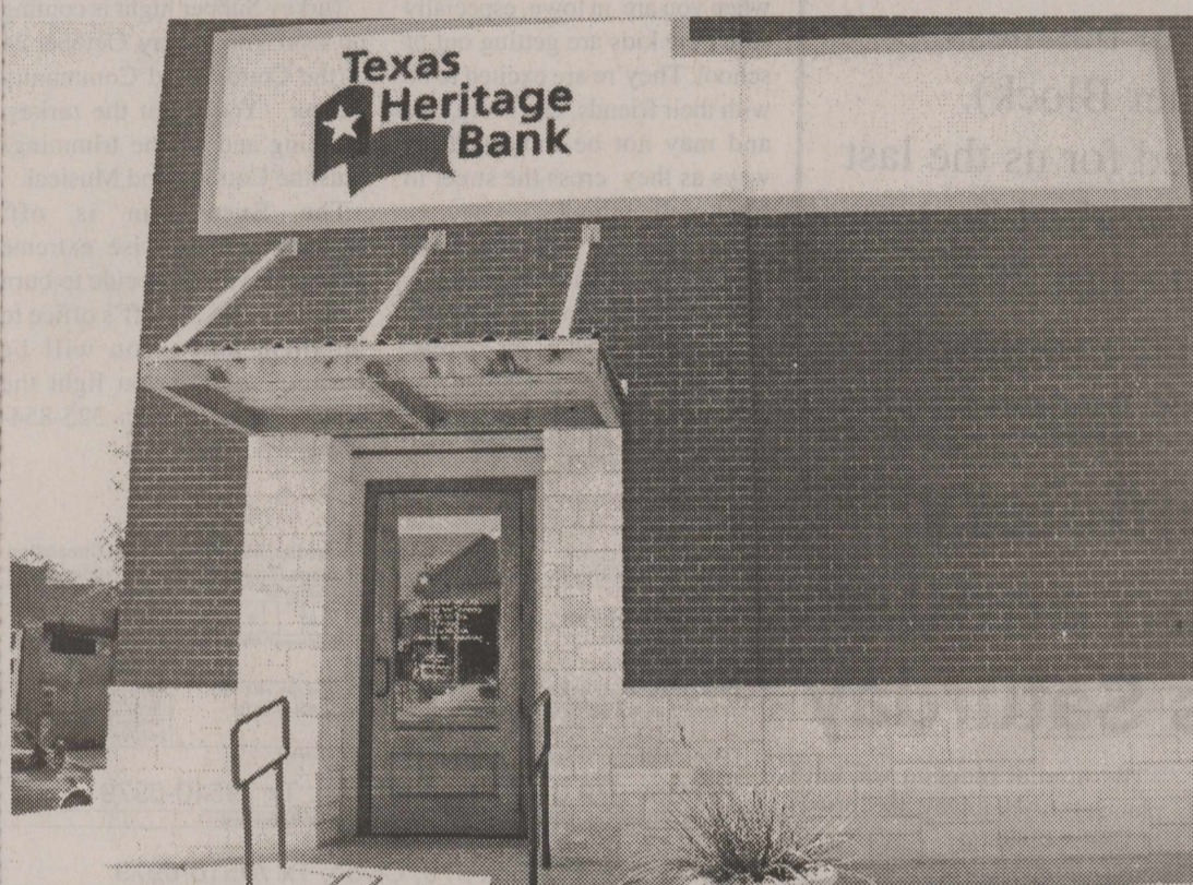
Texas Heritage after their exterior remodel. They received a brick and stone that was overlaid onto the top of existing brick. They also received a new awning.
