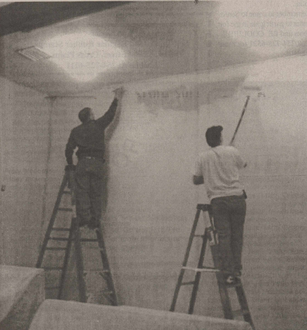
PAINTERS WORKING ON THE INSIDE.
