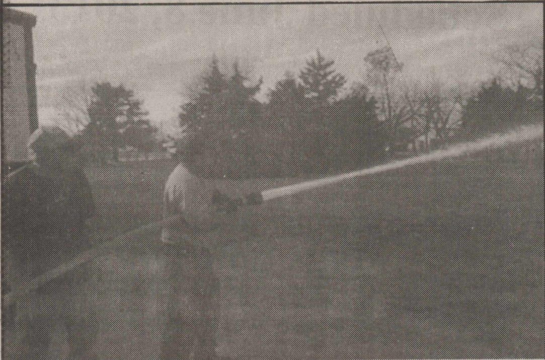
Firefighters checking water pressure — Cottonwood Volunteer Fire Control firefighters Jim Grindstaff, left, and Roger Hinkle, right, test the water pressure after the installation of the new pump and motor on Brush Truck No. 2
