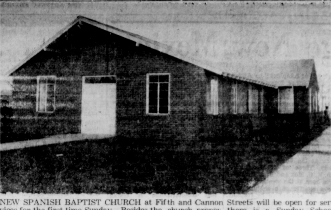
NEW SPANISH BAPTIST CHURCH at Fifth and Cannon Streets will be open for services for the first time Sunday. Besides the church proper, there is a Sunday School nursery and several other rooms. The Rev. N. E. O'Neill, who has been conducting Spanish Baptist services at the old location, is the pastor at the new church. (Advocate Photo)
