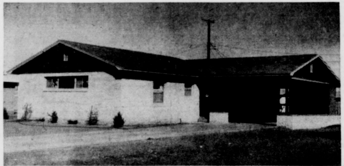
Above is the residence of The Charles Bruces at 1404 Hermosa in the Barnett Addition.
