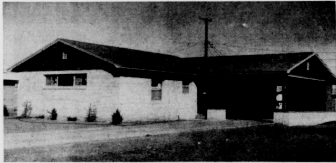
Above is the residence of The Charles Bruces at 1404 Hermosa in the Barnett Addition.
