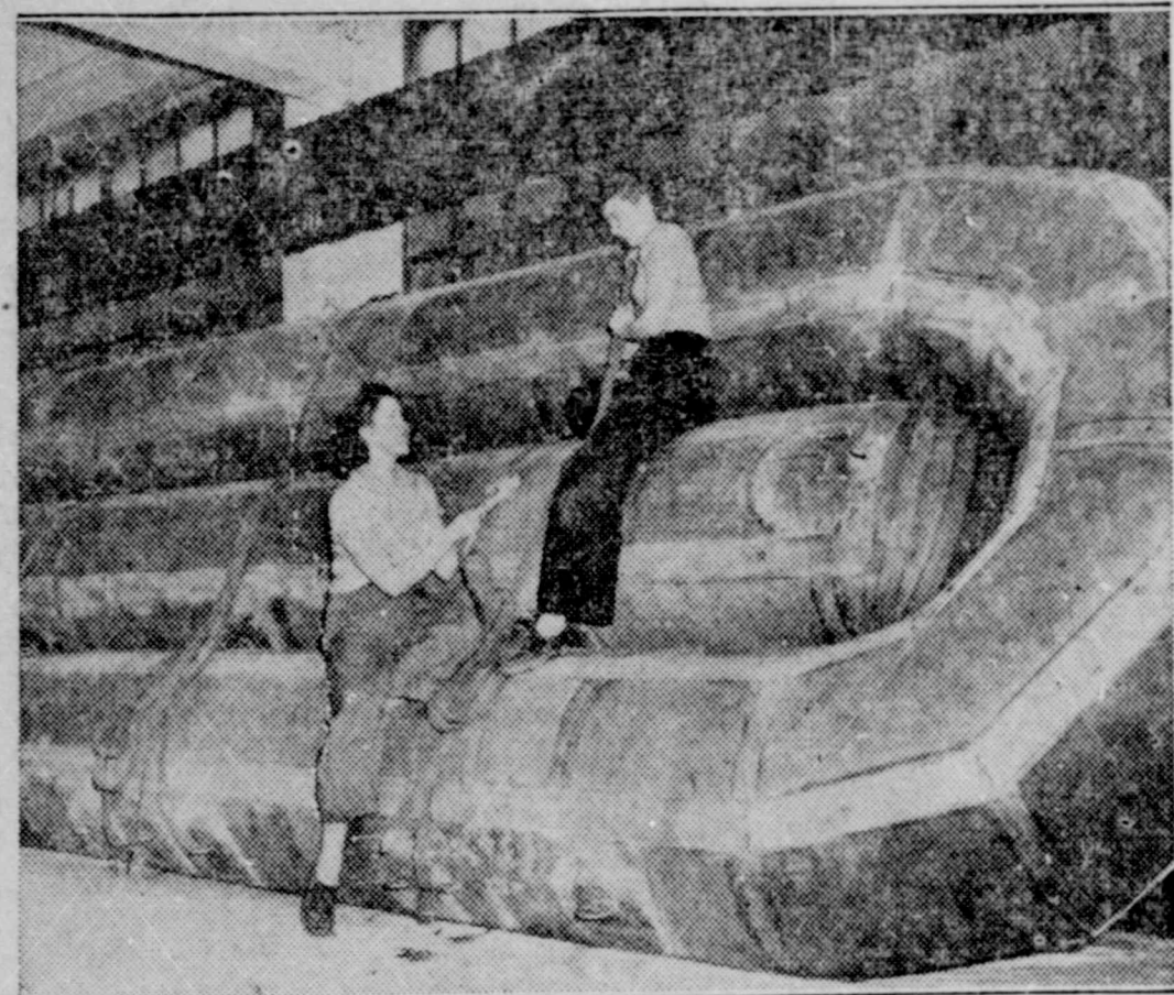
Massive rubberized cotton pontons like the one above aid in giving added mobility and striking power to U. S. armored forces. By the use of such pontons with heavy steel treadways, new armored force bridges can be erected faster and carry heavier loads than any other military bridge in existence.
