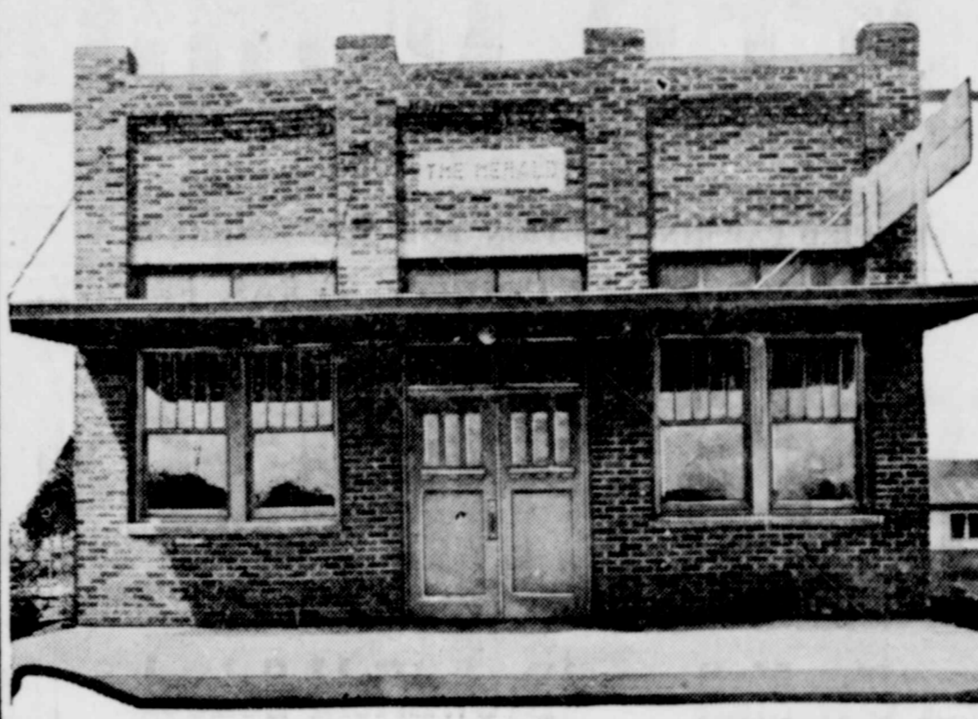
Here is a likeness of the present plant of the Herald. Constructed of brick and concrete, size 25x60 feet, can be enlarged to 50x140 feet with lots owned, but we don't expect to see this done—soon.
