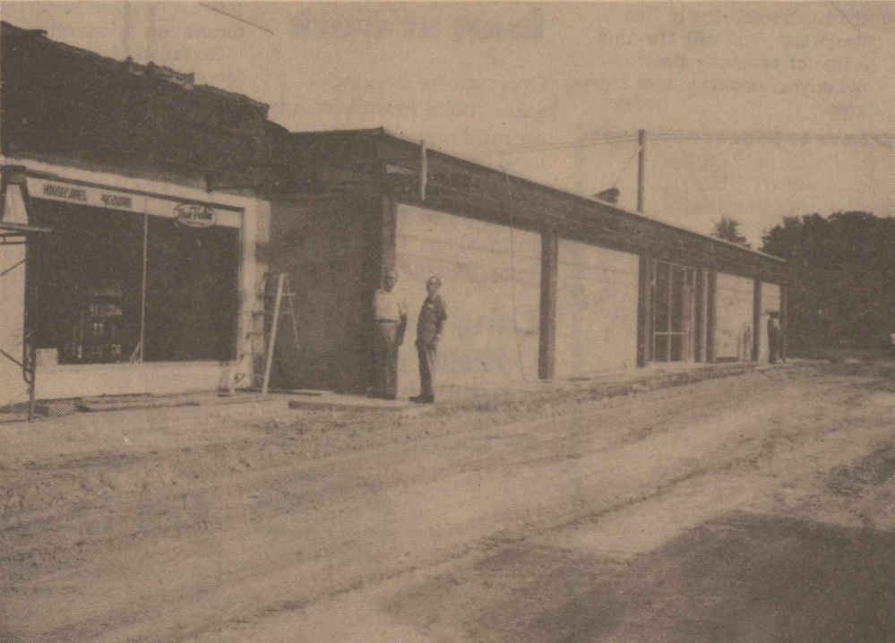
NEW ADDITION TO SOUTH TEXAS LUMBER CO. -- Work is progressing on the new addition to the company located at the intersection of highway 163 and I-10 in Ozona. The new addition will more than double the space of the present building. Here W. H. Whitaker looks over the expansion project with Arthur Madden, representative of one of the companies South Texas purchases materials from.
