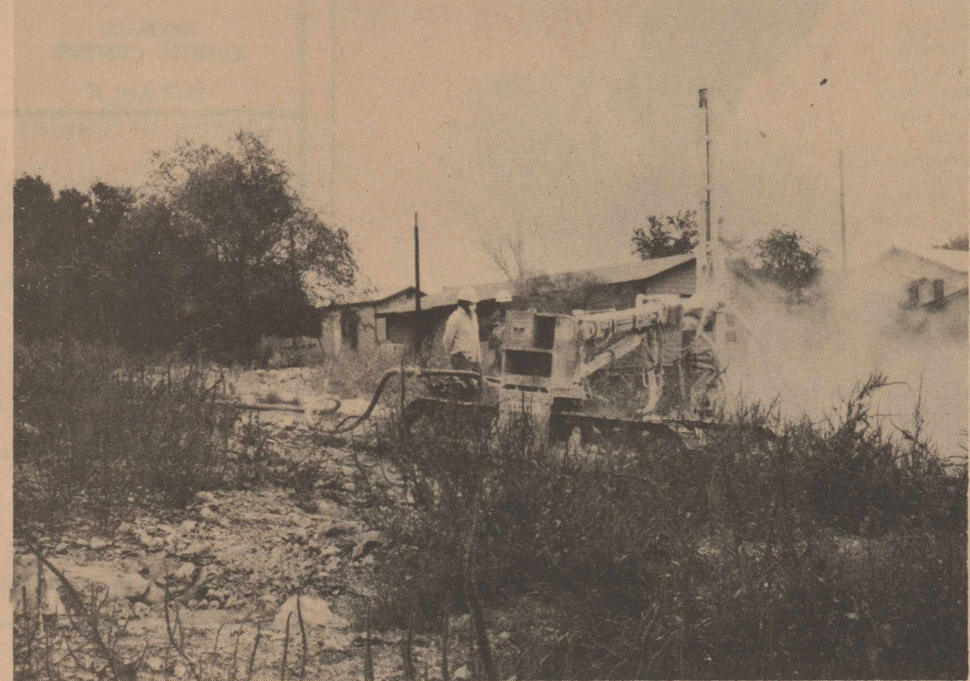
GETTING READY FOR THE DYNAMITE CREW -- This giant drill, operated by an air compressor, was at work Monday preparing for the blasts which will make the cut for IS 10 through the south part of Ozona. Blasts usually go off at noon and again at 6 p. m. Two Zachry Co. men are operating the drill.
