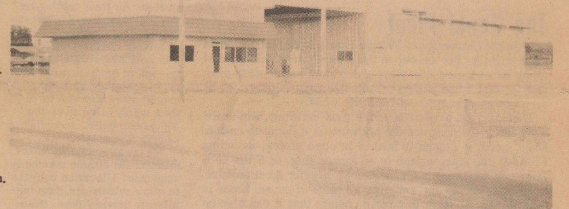
ALL FINISHED BUT THE FINISHING TOUCHES is the new County Maintenance Department. Paving around the building has not been completed, but other than that and a few minor fixins, the county crew should be able to move in soon. The handsome new county maintenance home is located north of Ozona on Hwy 163 across from the Highway Department.
