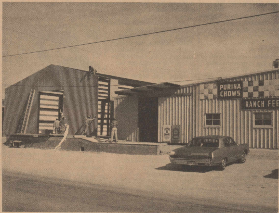
MORE WOOL-MOHAIR STORAGE space will be provided by this 7,200 square-foot addition to the Ranch Feed & Supply Co. warehouse here. The addition will be 60 by 120 feet built on the north side of the company's present building. The new building will be somewhat higher than the existing building, affording space for higher stacks of wool and mohair. A concrete dock in the front and back will afford ease in unloading or loading trucks. Lilly Welding & Construction Co. is building the all steel structure.
