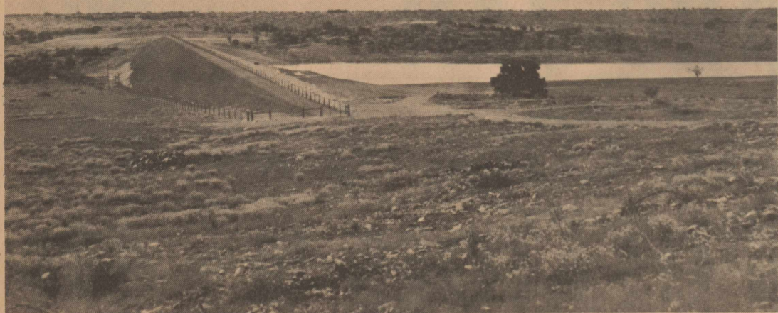
A FLOOD CONTROL DAM at work. The small lake of water is being held up by this flood control dam just north of Ozona. The picture was taken in 1958. Had just two or three such dams been in operation on the watershed, the damage in Ozona would have been only minimal in the 1954 flood. The dams hold up and permit an orderly flow of flood waters, preventing the downrush of the entire run-off from flooding rains.
