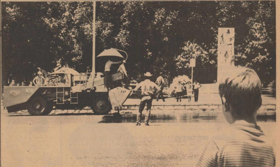
ROAD CONTRACTORS applying a seal coat surfacing to U. S. 290 made short work of the project in downtown Ozona. With multiple units at work, simultaneously applying hot asphalt and gravel and spreading and rolling new surface, the crew
