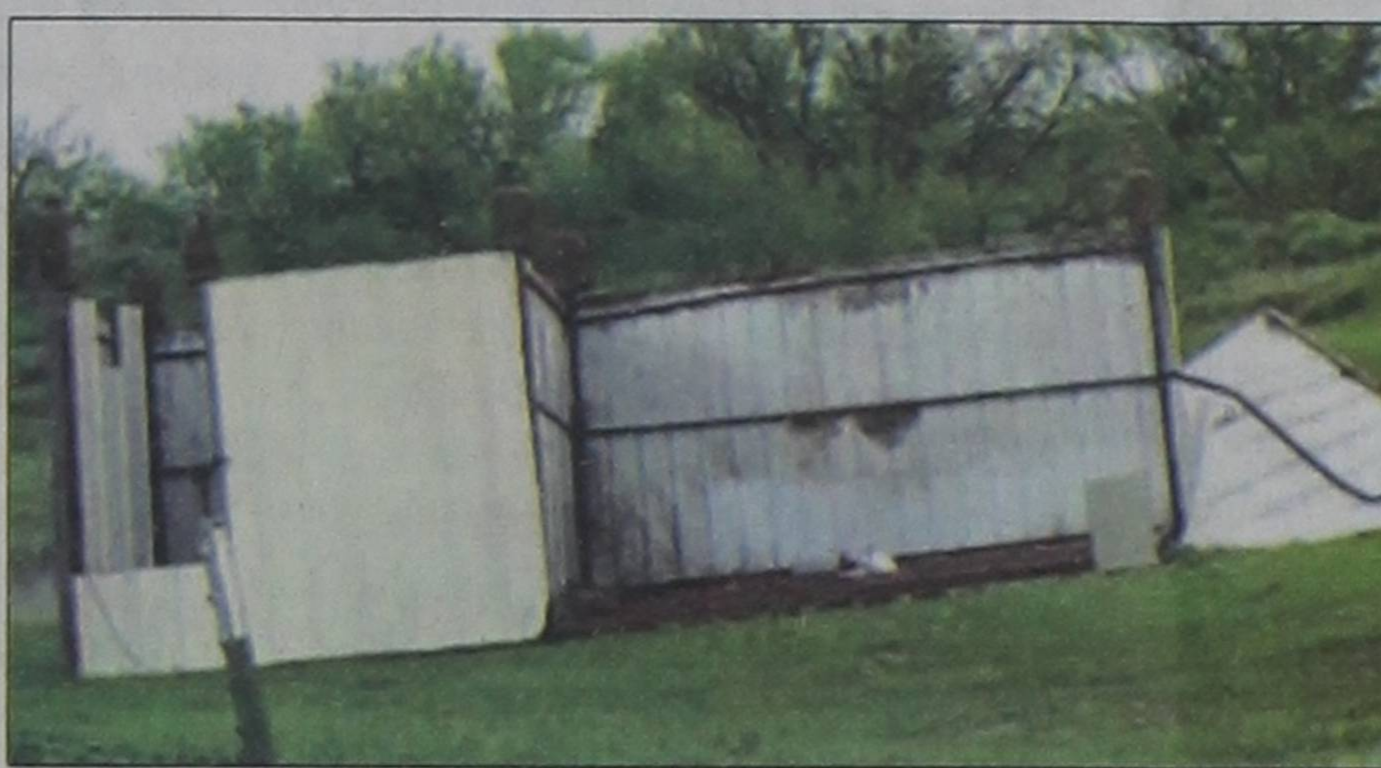
A 20' x 30' barn belonging to Lon and Nicki Adams was pulled up from its three-foot deep footings thrown over on its top during last Saturday's tornado.
