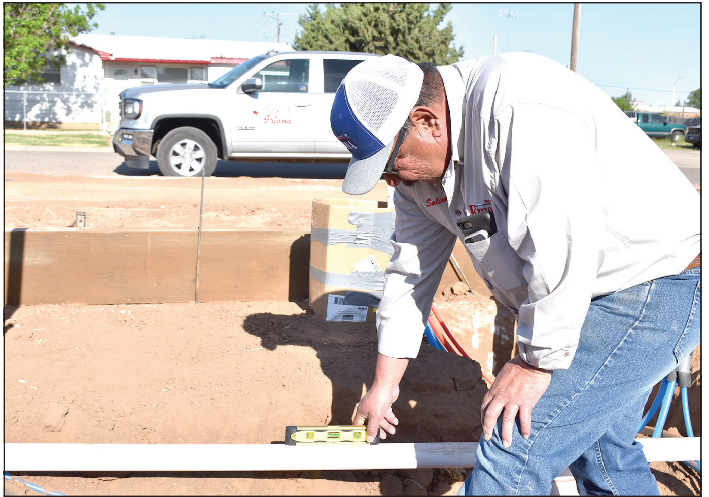
Public Works Director Salvador Garcia inspects work being done in Phase 1 of the new housing project at 6th and Ashland. The new triplex and quadplex residential properties are scheduled to be completed near the end of October.
