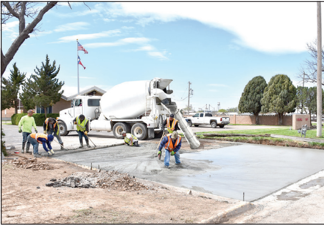
In the photo above, Bermea Construction, Inc. employees are installing a new concrete driveway at the Friona ISD administration building. The entrance was also widened to allow for easier access to the facility. In the photos below, construction has begun at the various school campuses.
